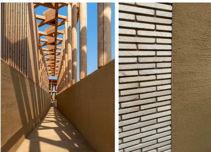
left: Designed for deconstruction Photo: Josef Sindelka / courtesy of Atelier Brückner right: Recycled local brick / clay from Awajishima Island, Japan
